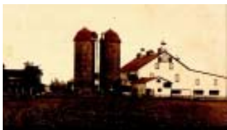
Millbrook Playhouse Converted Barn
